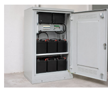
Demo battery backup
